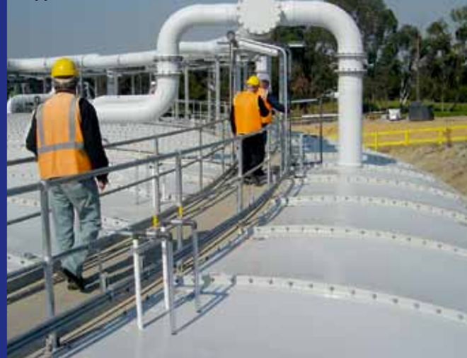
Gippsland Wastewater Treatment Plant
